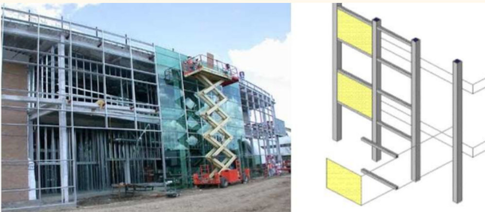
STICK-BUILT CURTAIN WALL INSTALLATION EXAMPLE
