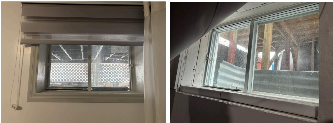
Windows at the basement bedroom #2 and mechanical room, respectively.
