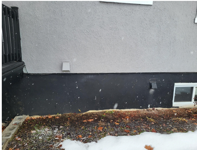
Cement parging located at the front side of the house.
