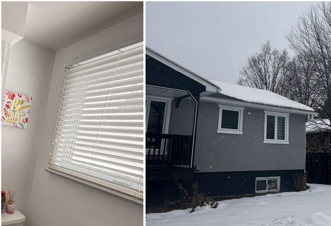
Windows from the main (upper) bathroom (left picture), and right-most window for the upper bedroom (right picture, interior view is unavailable due to privacy).
