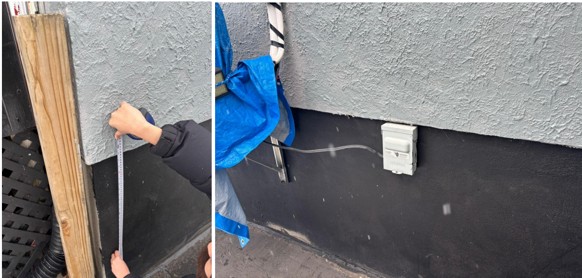
Cement parging located at the east side of the house.
