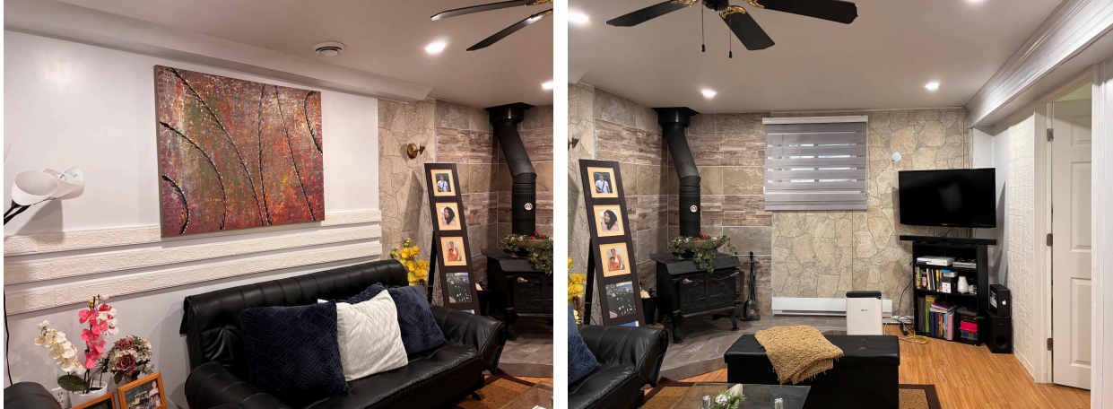
Fully finished interior wall and completely furnished room
